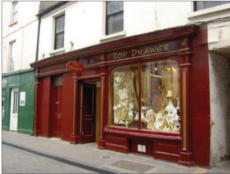
Figure 10. 2005 photograph of shopfront before closure of basement hatch to central panel beneath shop display window
