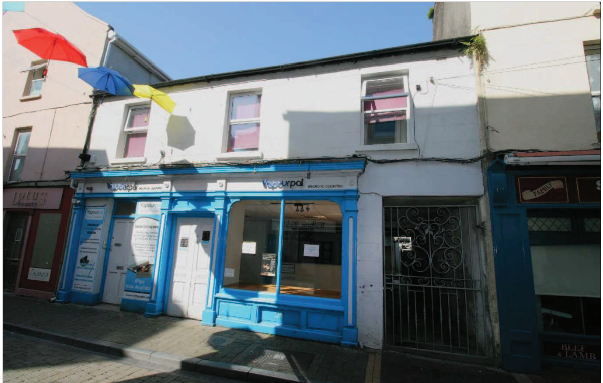
Plate 1. South façade fronting onto Mitchell Street with gated entrance to rear laneway on east side of front elevation.
