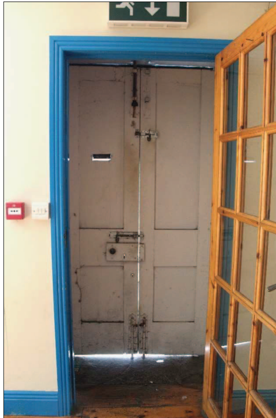
Plate 11. Detail of early to mid twentieth-century timber panelled entrance doors with modern glazed lobby door
