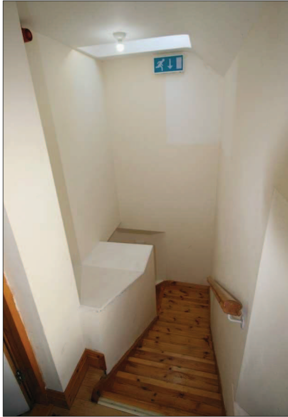
Plate 17. Modern timber staircase at west side of street-fronting building from first floor-level
