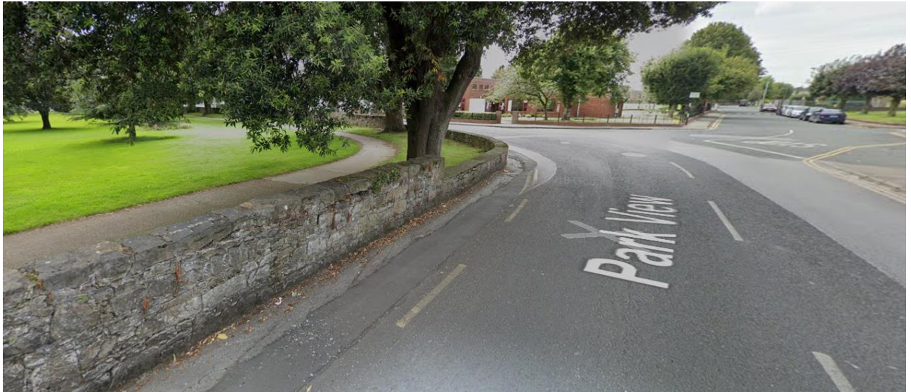
Figure 3.2: Existing tight bend and roadside walls on R697 Park View road.
