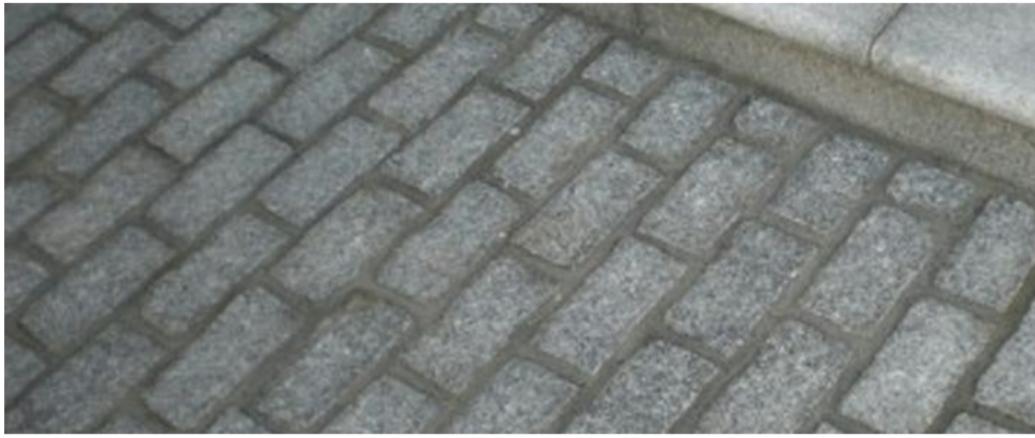
06 Carriageway, Feature Areas L902 Mid-grey flamed granite
