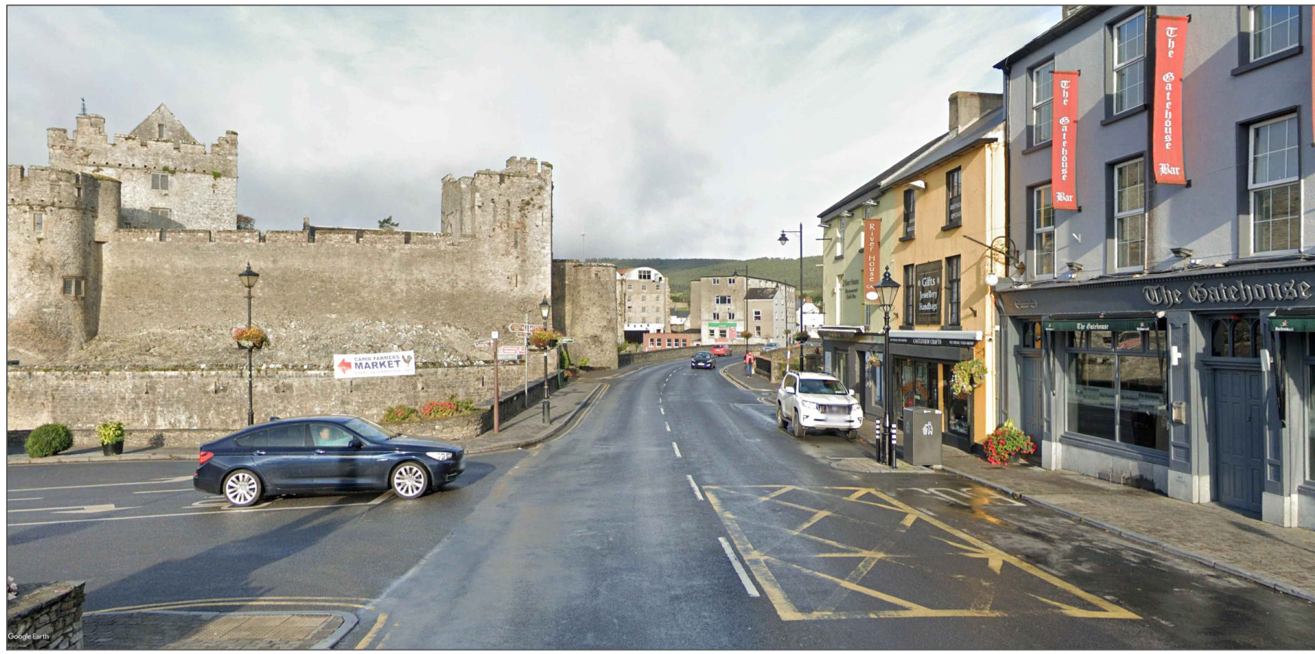
Castle Street: As Existing
