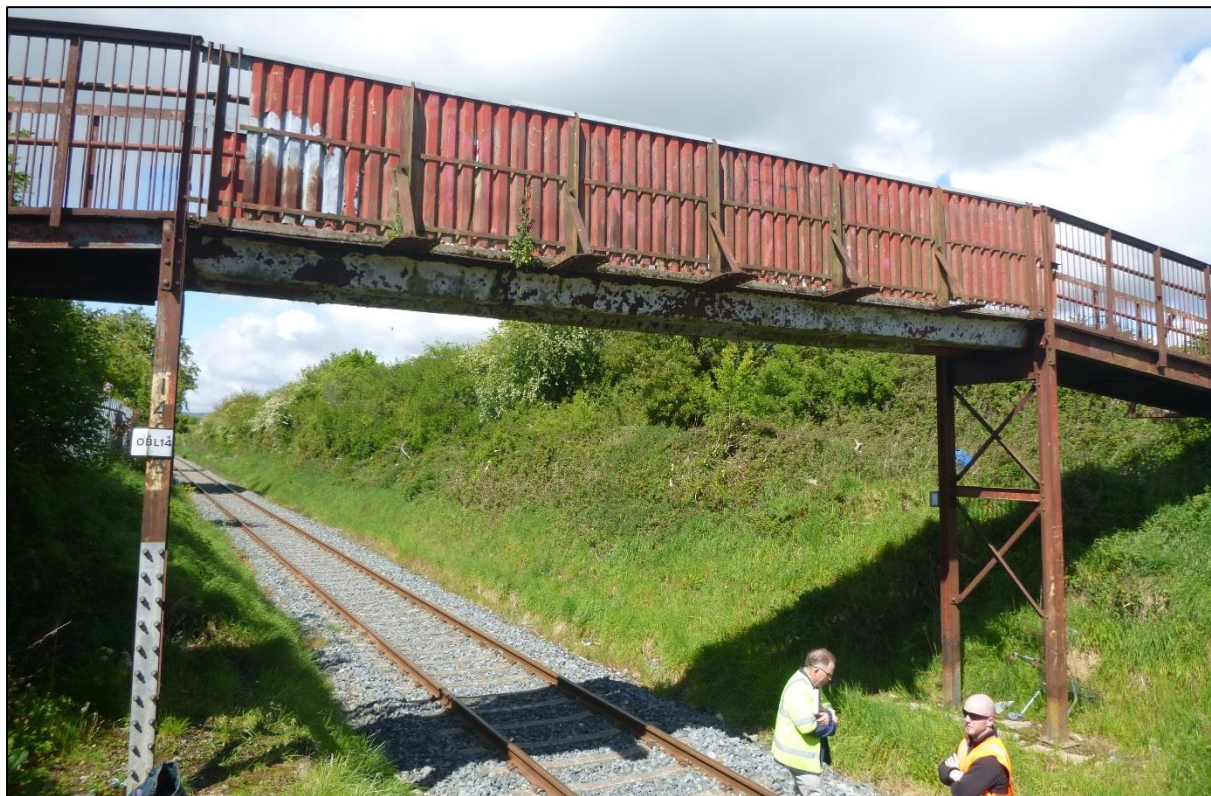
Figure 2-1: View of Existing Bridge Looking West
