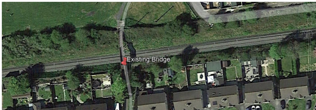
Figure 2-3: Aerial view of Existing Bridge
