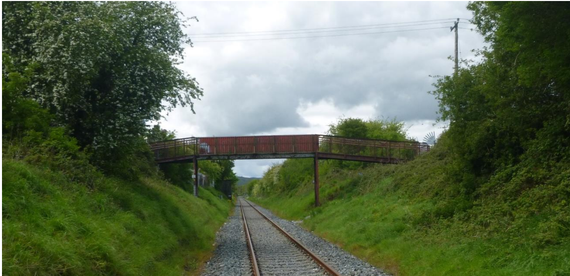
Plate 4-1: View of existing pedestrian bridge with embankments
