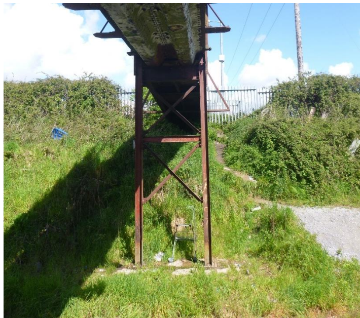
Plate 4-2: View of underneath pedestrian bridge with embankment.
