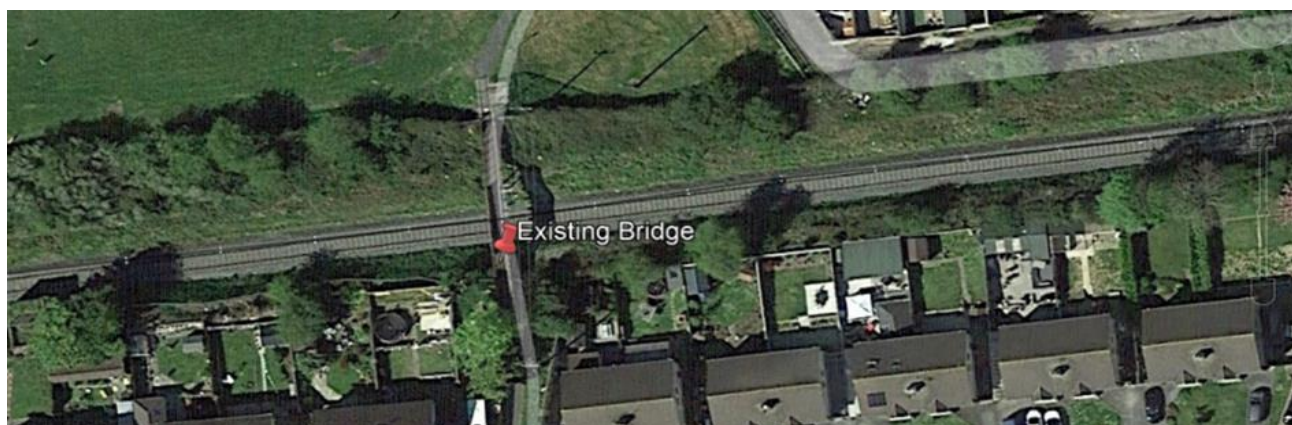
Figure 4-3: Aerial view of Existing Bridge
