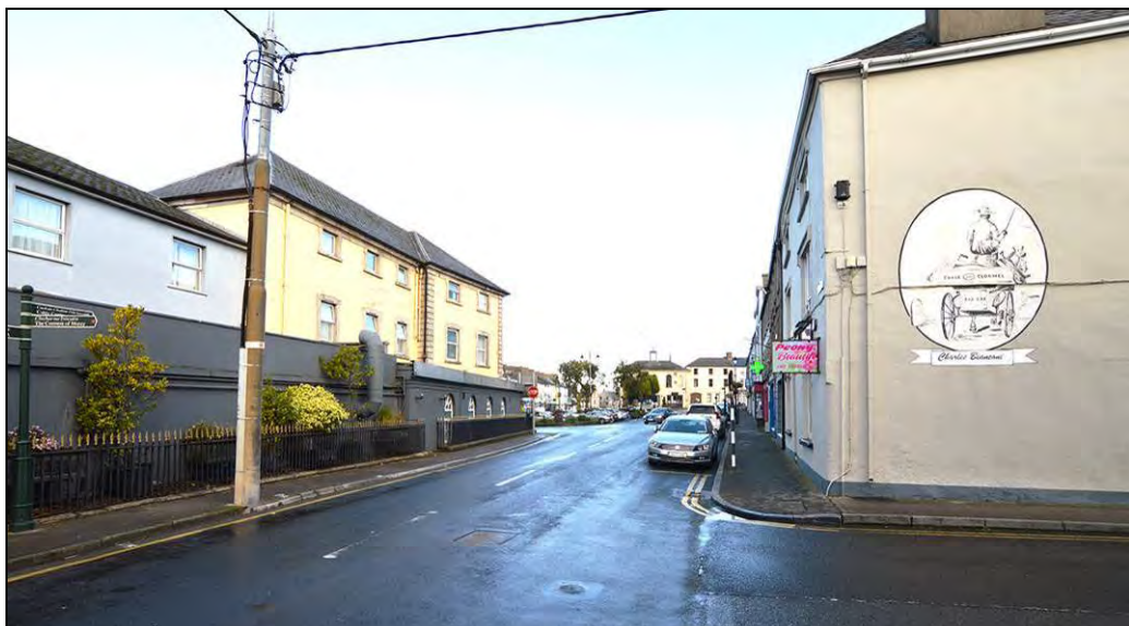
Photograph 10: View of works area on St. Mary's Road, looking north to the Square.
