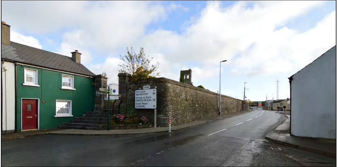
Photograph 1: St. Mary's Church and Graveyard, the medieval parish church of Cahir, at the start of the works at the east end of Old Church Street. The double bellcote that tops the west gable of the church can be seen breaking the top of the wall.
