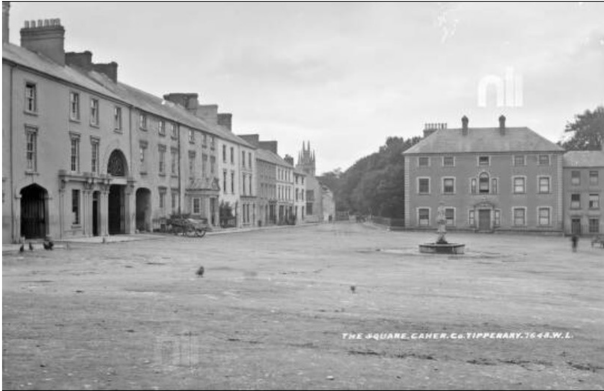
View to south of the Square, showing Cahir House and the eastern side of the square.
