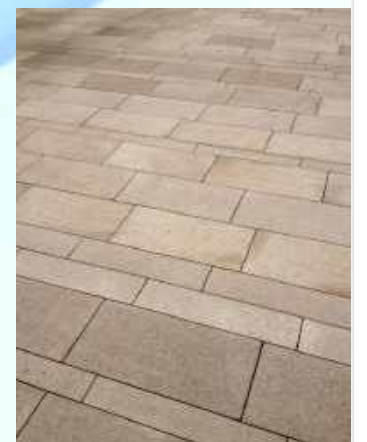
High quality paving
