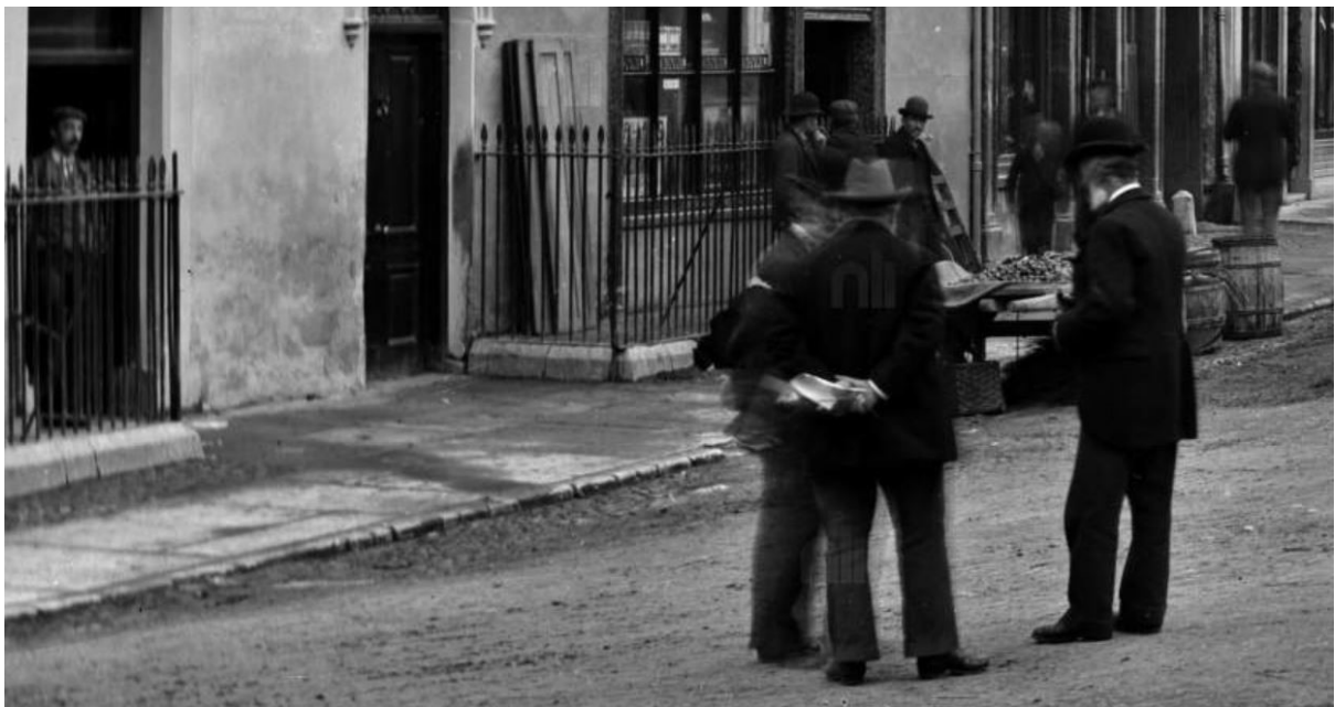
Details of paving and railings to the Square - flagged pavement, cobble stone drains, spearhead railings set in limestone, limestone kerb stones.
