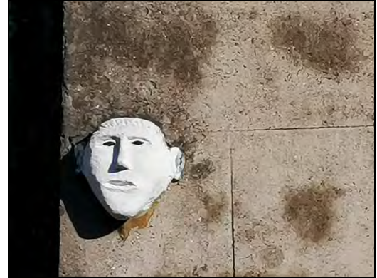
Photograph 18: 15 th Century carved stone head inserted in the elevation of 7 Castle Street.
