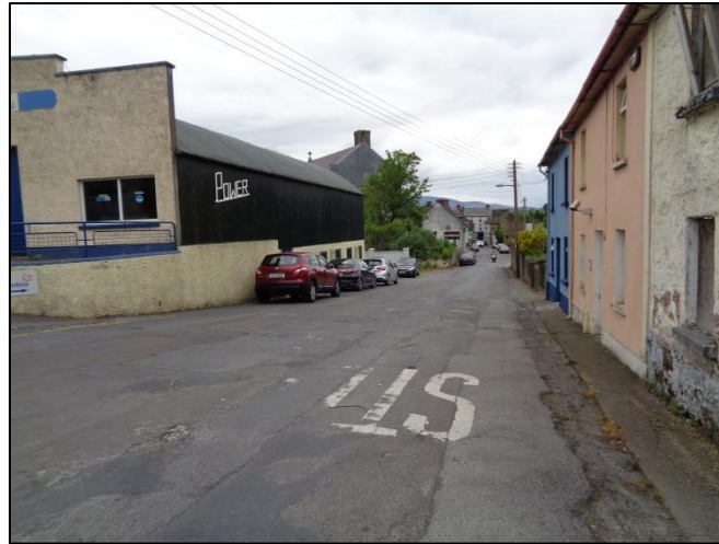
Pl. 1. Looking Northwest along Waterford Rd.
