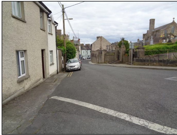
Pl. 11. Looking East along Friar St.
