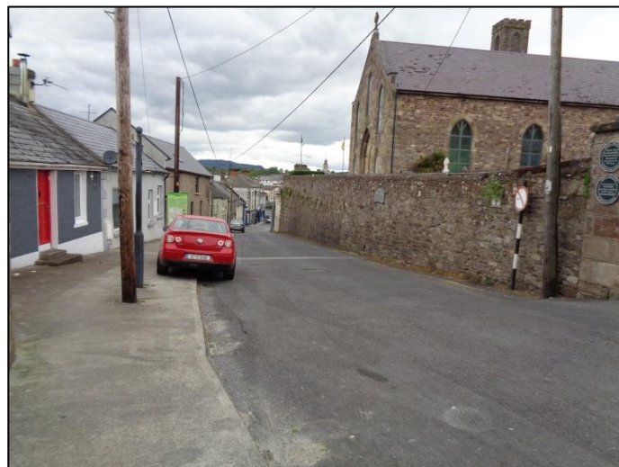
Pl. 8. View of St. Molleran's RC Church and Stone Boundary Wall.
