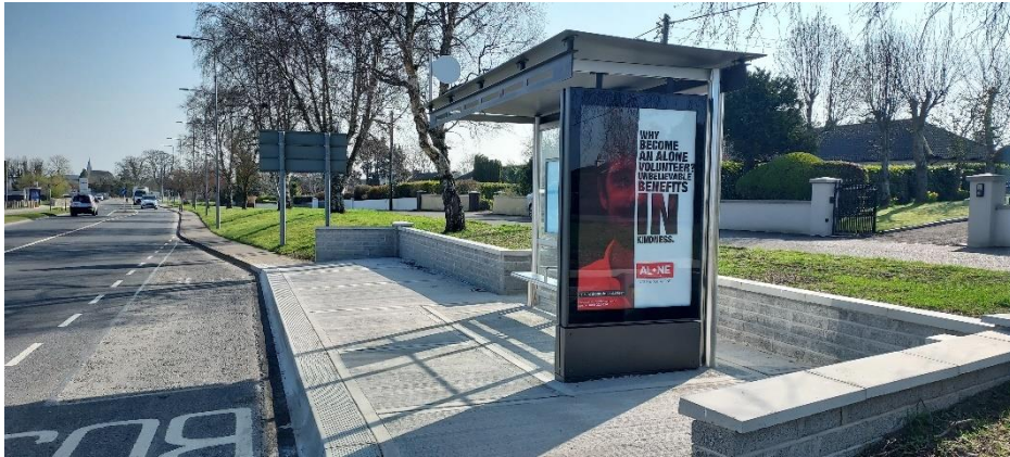
Figure 6.13 Example – Bus shelter provided at Springfield Retail Park
