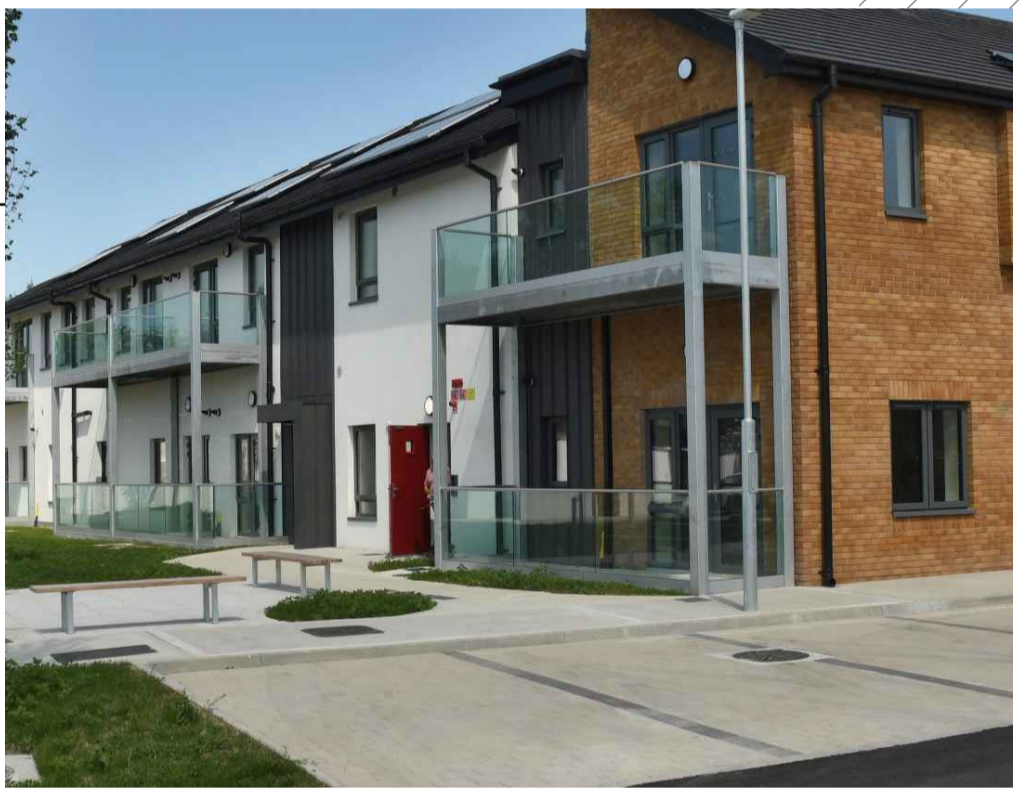
PRECEDENT IMAGE OF PROPOSED 1.1M HIGH TOUGHENED GLASS GUARDING WITH HOT DIP GALVANISED MILD STEEL BASE RAIL. TO BE USED TO AROUND PRIVATE COURTYARD ONLY.
