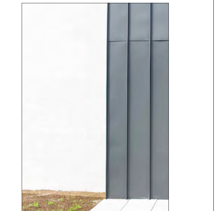
Precedent image of Proposed White Plaster Finish with Selected Colour Standing Seam Aluminium Cladding Panels Finish.
