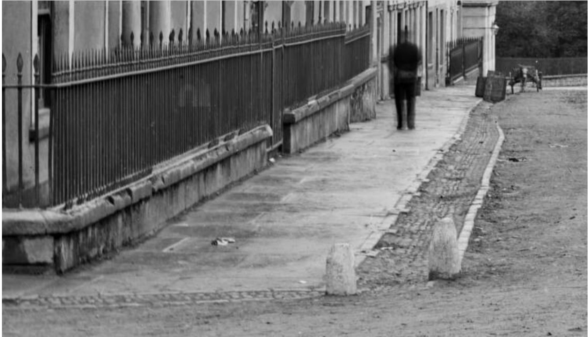
Spear head railings, cobbled drain, flagged pavement, limestone kerb stones and jostle stones to corner – details from c.1900 photograph of Bridge Street (NLI)
