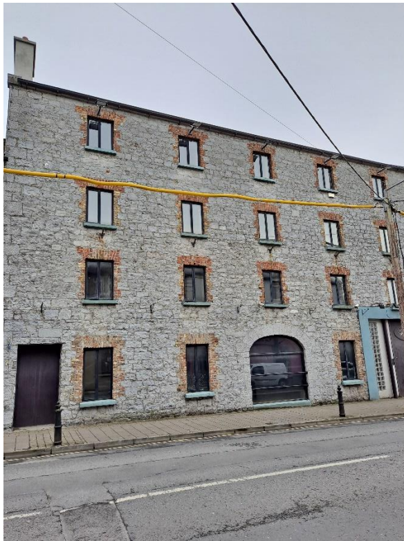
Plate 14: Building CHS 7 from opposite the road.
