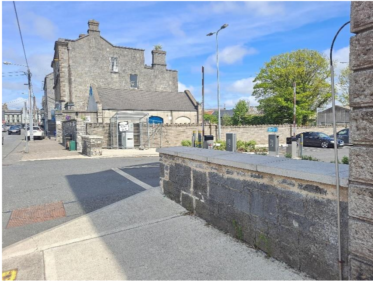
Plate 17: View northeast of new Council carpark off Slievenamon Road between CHS 8 & CHS 10.
