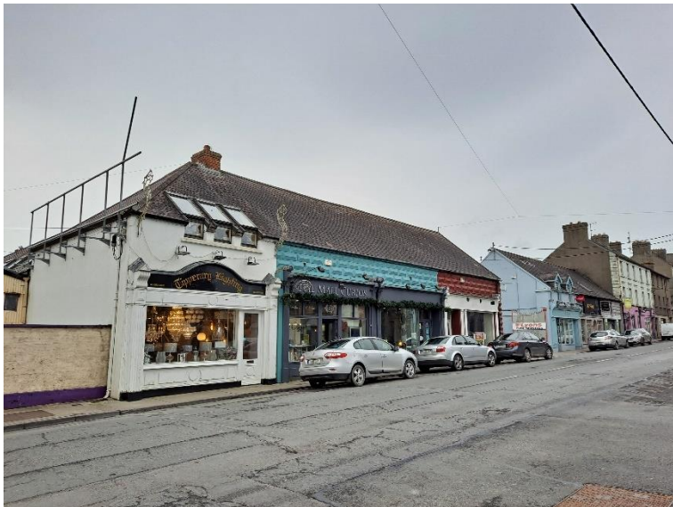
Plate 20: View northwest of Slievenamon Road opposite building CHS 10. Roadside boundary wall of CHS 9 at left.
