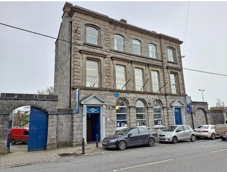
Plate 16: Building CHS 8 showing original ashlar limestone work with carriage archway at left & blind arch at right. This was the location of the National Bank on what was then known as Bank Street.
