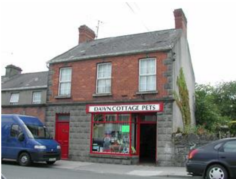
Plate 39: Building CHS 24 on the west side of Slievenamon Road beside CHS23.
