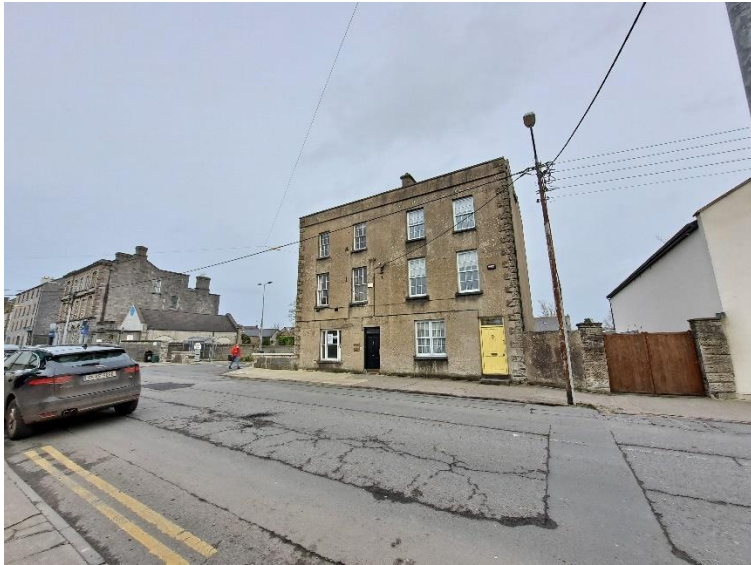
Plate 22: View east of buildings CHS 10 & CHS 11. These buildings marked the approximate end of Bank Street/The Middle Mall, south of which was largely agricultural land on both sides of the road.
