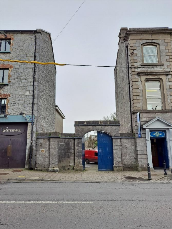
Plate 15: Junction of buildings CHS 7 & CHS 8 showing original carriage archway.
