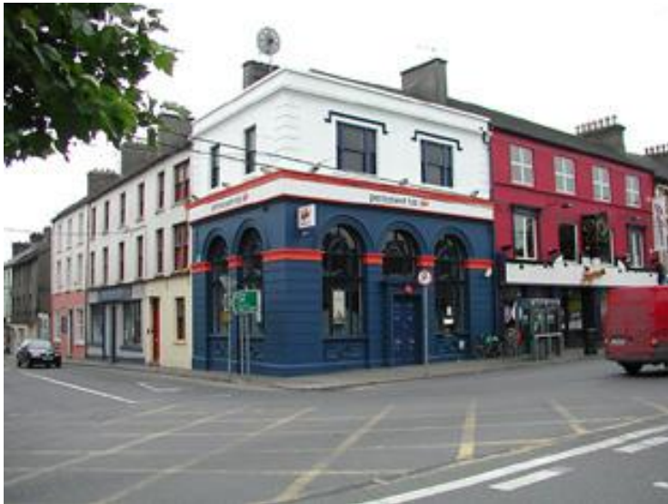
Plate 8: CHS 4 looking south from Liberty Square.
