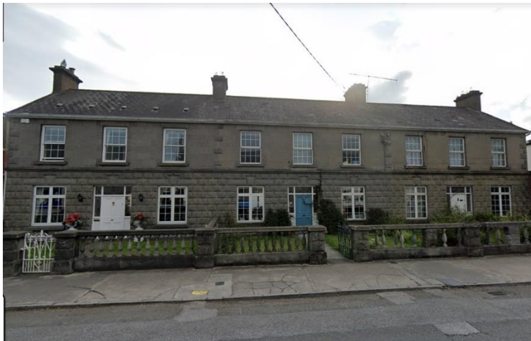
Plate 40: Terrace of three-bay two-storey houses CHS 25-CHS 27, on the west side of Slievenamon Road.
