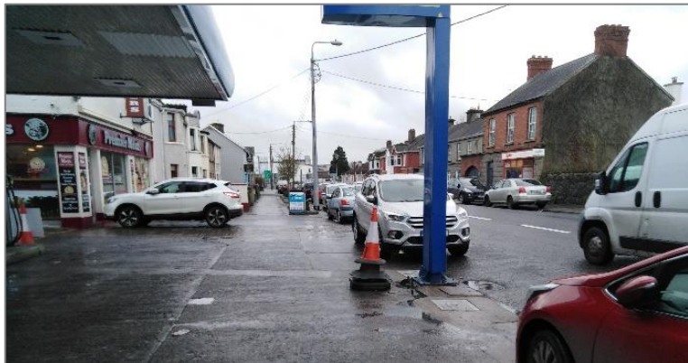
Lack of footway definition across service station forecourt and access points
