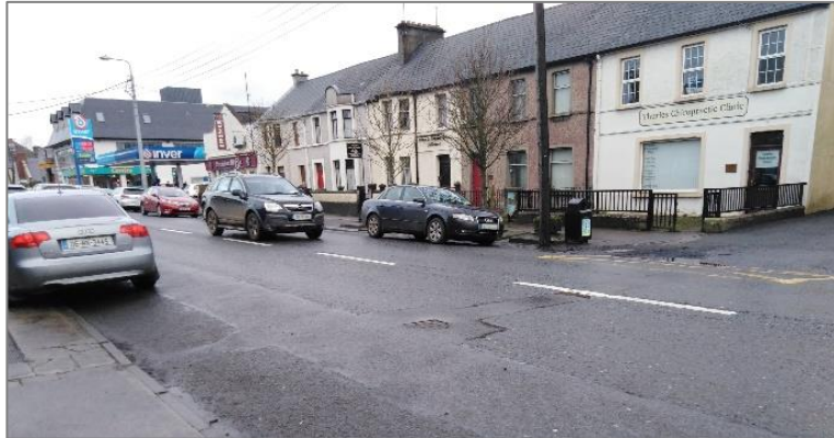
Wide road cross section in places (greater than 10.0m) with poor footway surface
