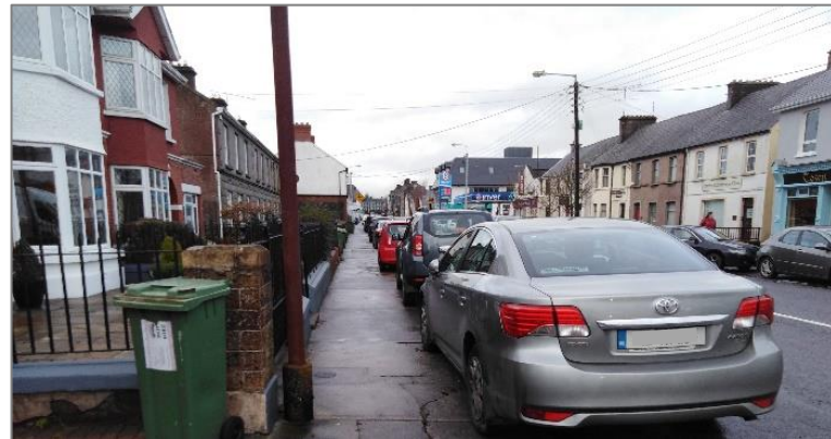
Illegal parking on footways causing obstruction and damage to surface
