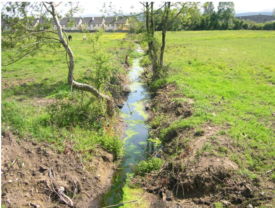
Photo 2: Drain upstream of culvert
