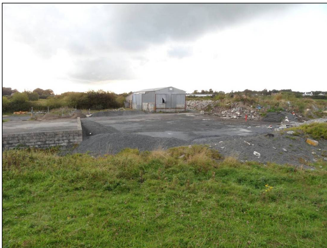
Plate 12 View of the old buildings and material storage on the closed landfill site.
