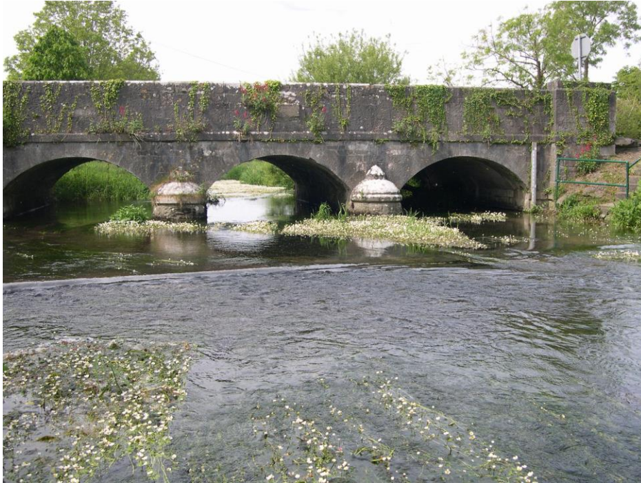
Photo 11: Downstream of Bansha Bridge
