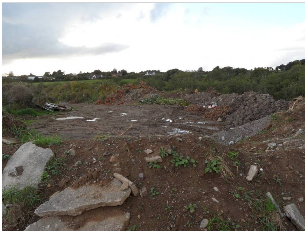
Plate 14 To the north of the fenced compound on the landfill there is an area of freshly dumped topsoil, construction waste and vegetation. This is piled along the embankment at the edge of the swamp habitat.
