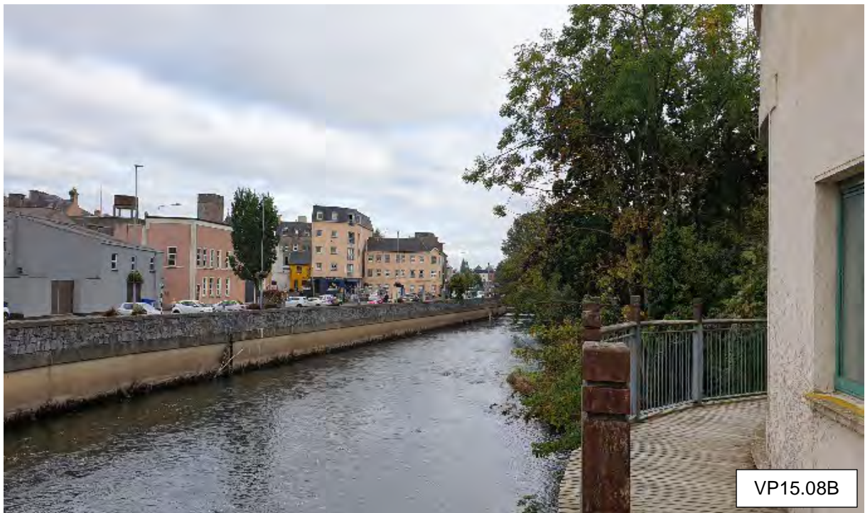
VP 15.08B From Hughes' Mill looking northeast towards Sarsfield Street junction off The Quay road, single tree at existing car park, and beyond the proposed location of North Bridge.
