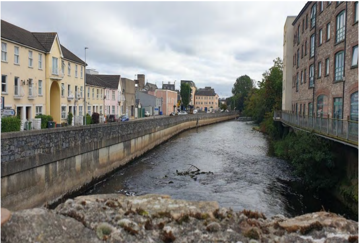
Image 15.4_01A, From the Old Bridge, the northern end of the bridge. Looking East (Existing view).
