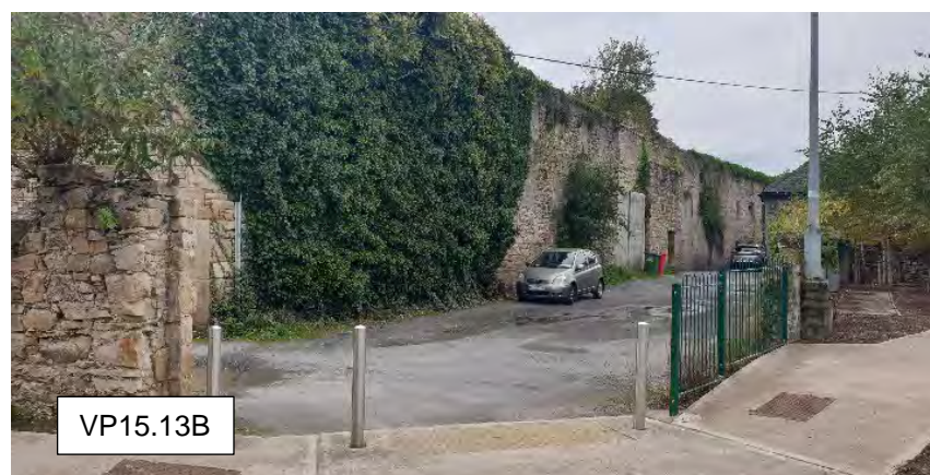
VP 15.13A & VP 15.13B Location of proposed shared entry point from the carpark to the access ramp to the proposed promenade (to the left of this view), to the Suir Island Gardens' entrance and onwards to Old Bridge via the existing narrow laneway.
