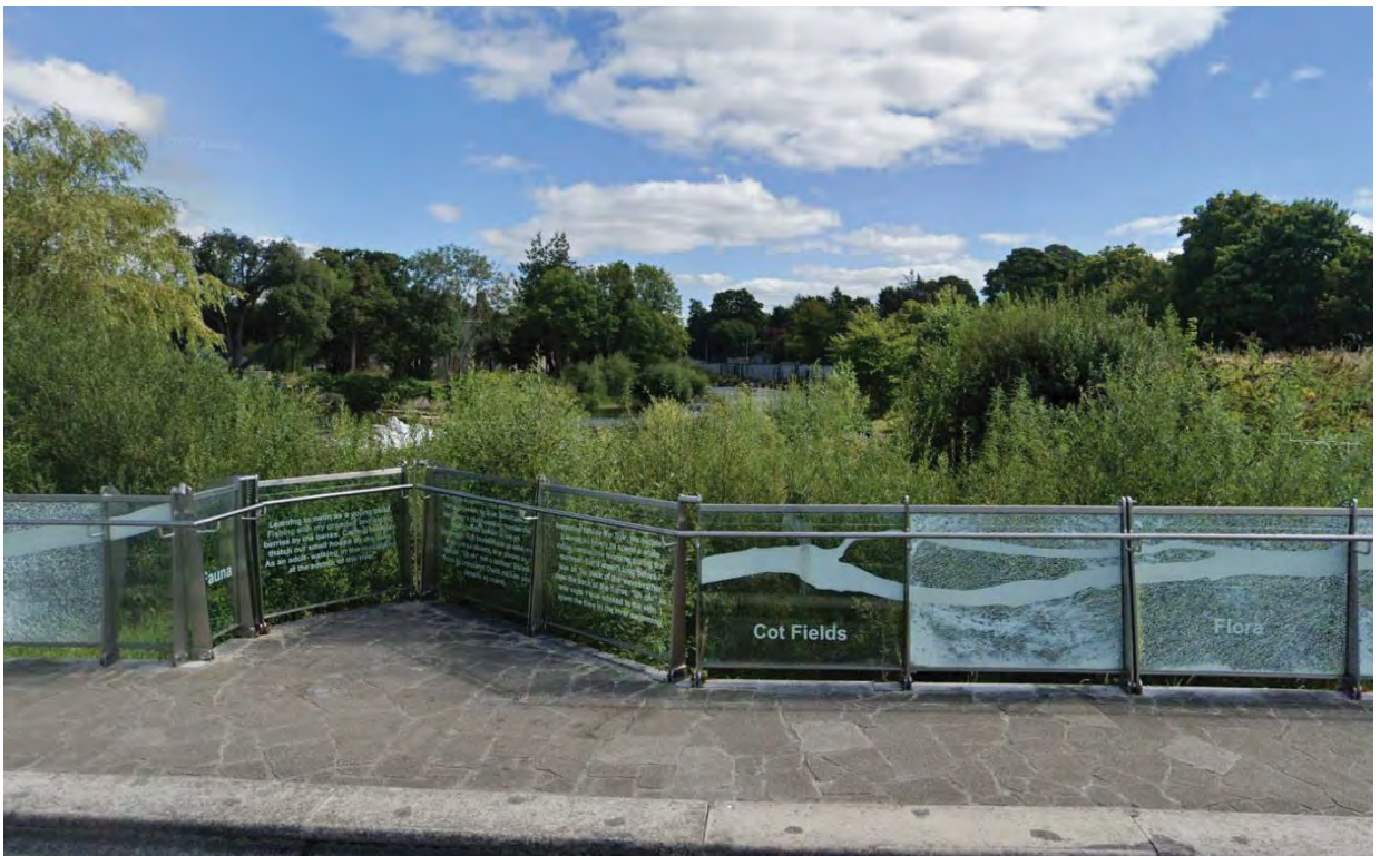
Image 15.4_02A, From the south end of Old Bridge looking east (Existing view).
