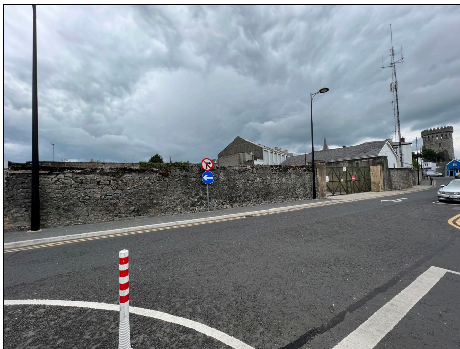
Plate 3: NE facing view of the yards stone enclosing wall from Emmet Place – note Nenagh Castle in the background.
