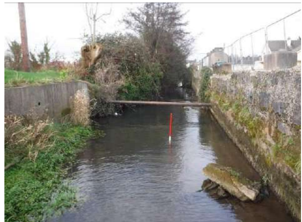
Plate 18 Area of deep water Chainage 2330, facing north
