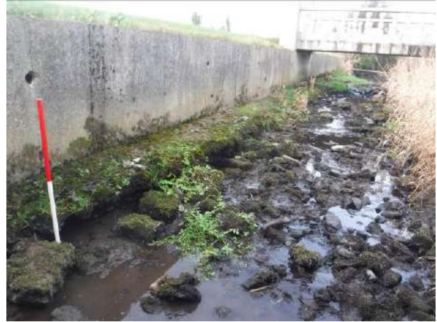
Plate 20 Concrete channel walls and concrete plinth foundation, facing northwest
