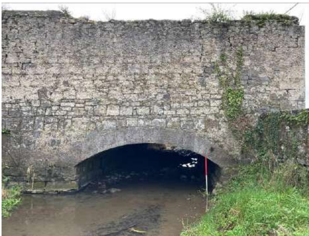
Plate 9 Large Stone Arched bridge/structure, facing south
