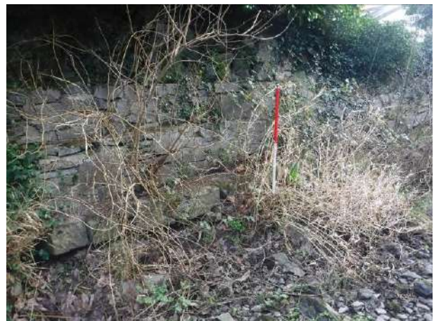
Plate 24 Channel Boundary Wall south of Small Bridge, facing southeast
