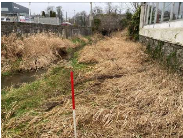
Plate 11 Overgrown area upstream from O'Dwyer's Bridge, facing north
