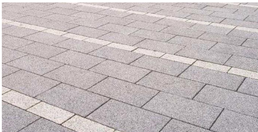
Figure 3-1 Surface Finish – Secondary Pedestrian areas
