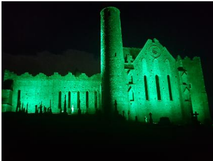
Figure 10 Rock of Cashel Colour Change Lighting System
