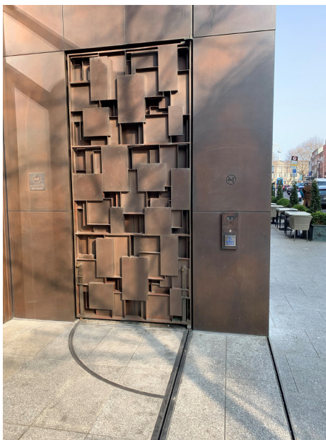
Design reference - recessed metal gate & track
