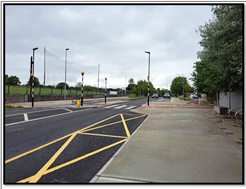
Figure 15: Segregated cycle track, uncontrolled crossing and cycle parking at N24 Pill Road.
