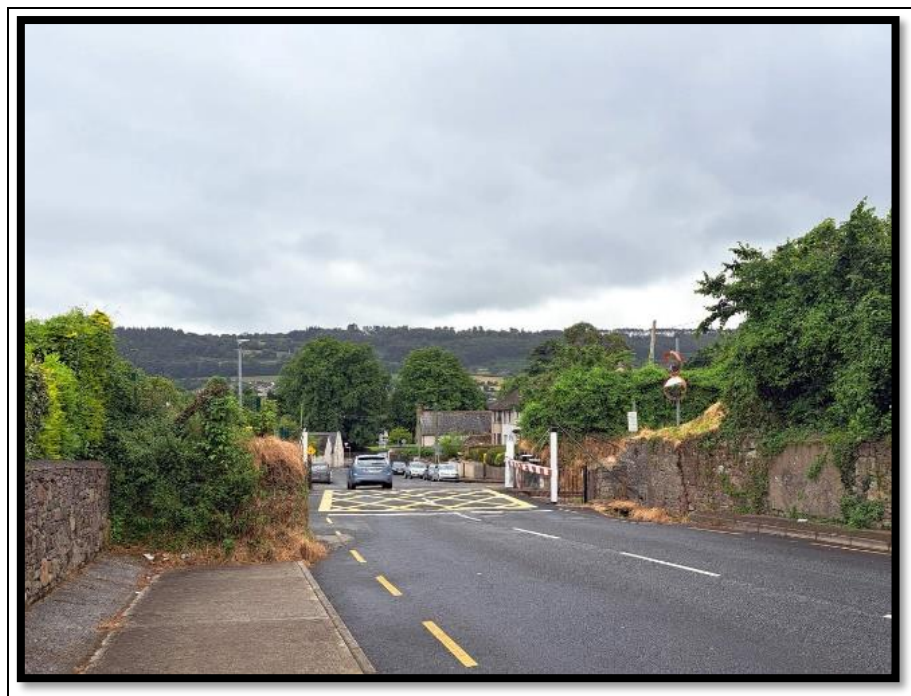
Figure 14: Level crossing on Cregg Road.
