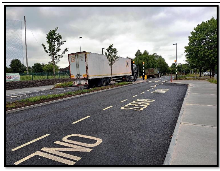
Figure 13: Active Travel Upgrade works on N24, Pill Road.
