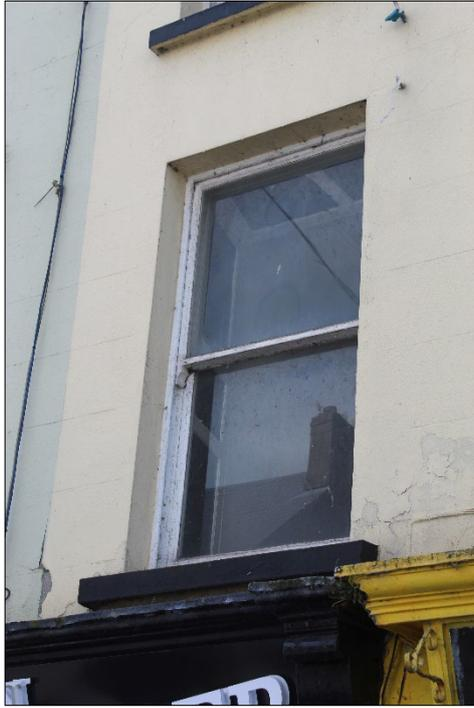
*Plate 11: Traditional timber sash windows with fine dimensions of glazing bars and mid-rails are possible to retain and refurbish as functioning, attractive features of a historic building. Specific moulded details of historic sash horns and frames contribute to distinctive character of ACA and are not well-replicated by mass-produced replacement windows.*
