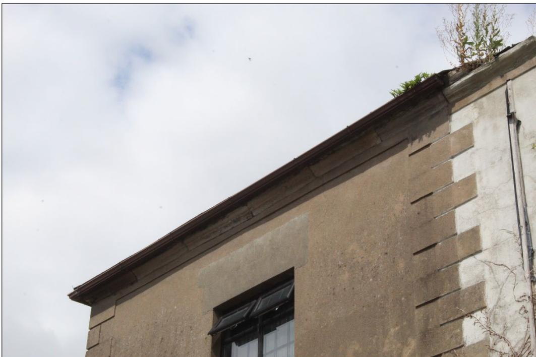
*Plate 14: Moulded stone, oversailing eaves cornices should be retained and appropriate, durable gutters should be fitted such that they do not cause damage or obscuring of such distinctive decorative features*
