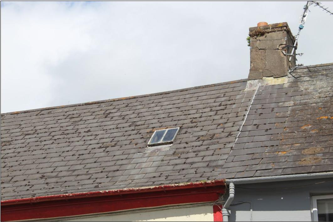
*Plate 15: Retention and appropriate refurbishment of traditional features such as natural roof slates, cast-iron roof-lights and eaves gutters as well as chimney stacks help to keep much of the traditional character of the streetscape intact.*
