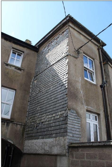
*Plate 17: Localised examples of traditional slate hanging, particularly on rear elevations and stairwells such as this, should be retained and conserved using appropriate lime mortar.*
