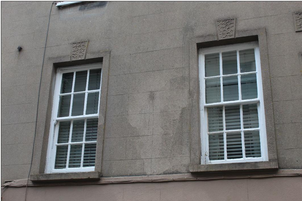
*Plate 12: Localised repairs to existing window frames and sashes, stripping back of built-up layers of paint and recoating, appropriate draft-sealing and renewal of cords, weights and fittings where necessary are encouraged and are eligible for grant assistance where available.*
