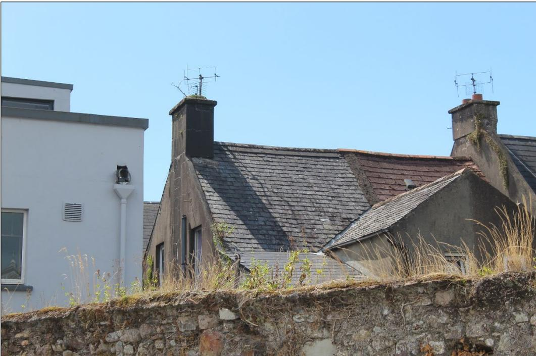
*Plate 16: Particular significance is attached to local materials such as Ahenny natural slate with any remaining examples of this conserved in an appropriate manner.*
