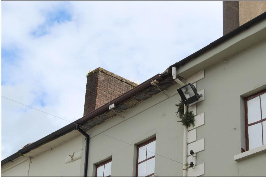
*Plate 13: Deep, overhanging stone eaves are a particular feature of terraced buildings in Carrick-on-Suir which should be retained and incorporated in redeveloped buildings.*
