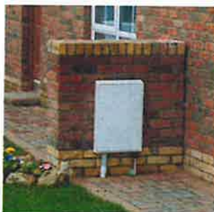
Domestic meter box
